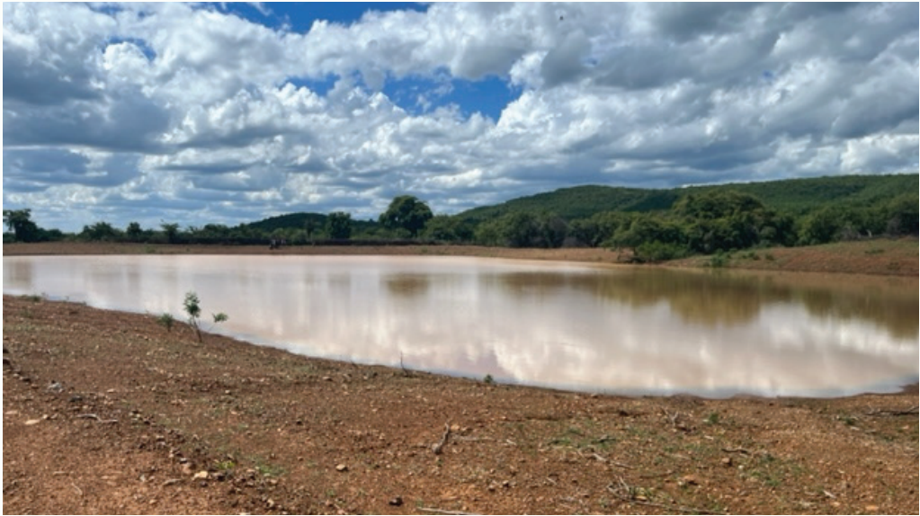
Cherumbo Water Pan after desilting collected water enough to serve the community.
